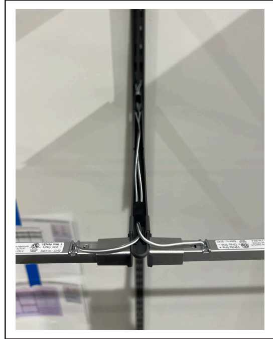
Position light, pushing one side in place. Lift other side up until straight. Magnet and tension rod will hold in place.
