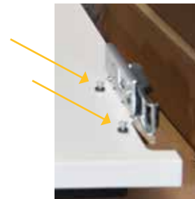
Dowel Holes in front of Suspension Brackets (#10)
